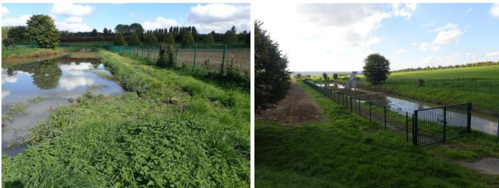
Figure 10 : Bassin 53030 (photos C.Adell © Egis, 09/10/15)
